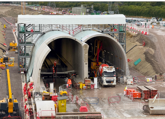
Concrete arrives underneath the arches. Photo: Murray Cooke.
