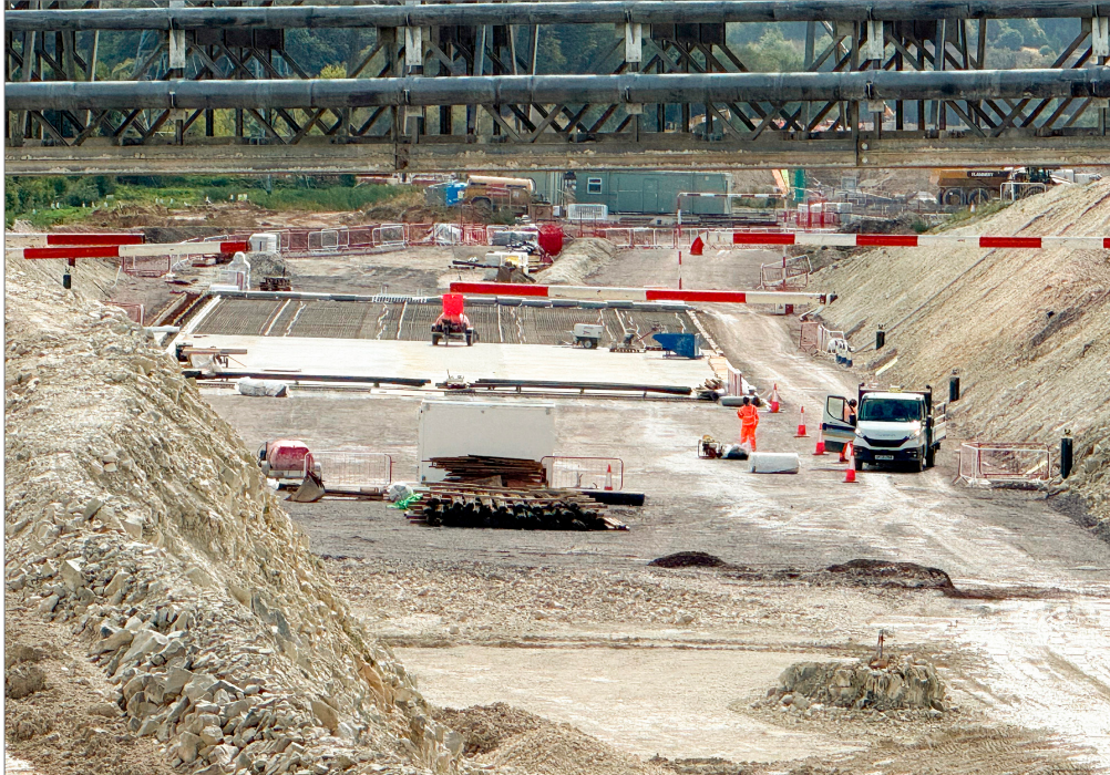
Green Tunnel phase 2 foundation slab being laid near Bacombe Lane. Photo: Murray Cooke.
